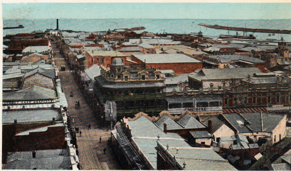
FREMANTLE, LOOKING WEST, W.A.
