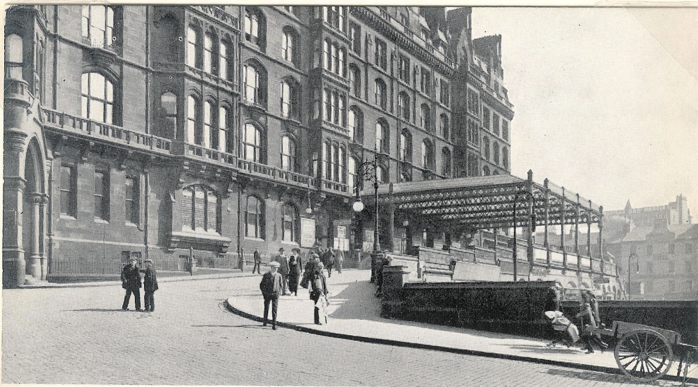
ST. ENOCH'S STATION, GLASGOW. "NONSLIP" STONE FLAGS—GRADIENT 1 IN 8. Supplied by "NONSLIP" STONE CO., Halifax, London, and Manchester.
